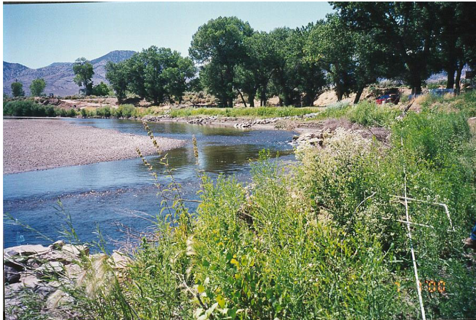
Figure 7. View upriver in August 2000, 21 months after installation of bioengineering treatments; the peaked stone dike with brush layering is shown in foreground
