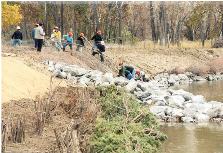
Figure 6. Three bioengineering treatments: (a) live willow clumps with a juniper tree revetment (foreground); (b) workshop attendees installing brush mattress with rock toe protection (middle of photo); (c) brush layering over peaked stone dike (far right of photo). Erosion control fabric with seeded riparian grasses appears on upper bank on left side of photo
