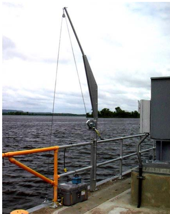
c. Hoist used to raise and lower test panels. The large gray box and the small blue box at base of hoist are the EESS’s power supply and control boxes, respectively.
