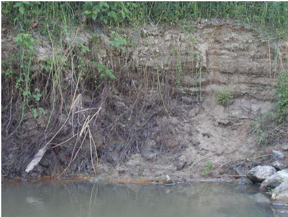
Figure 4. Reach 11, bank sample location next to bendway weir
