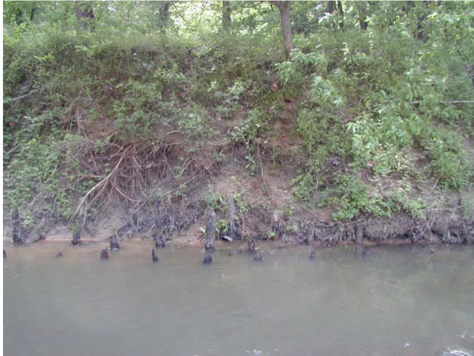
Figure 5. Reaches 6 and 7, willow post site, bank sample location
